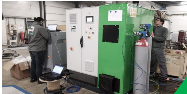
BIOGAS, H 2 and BIO-CH 4 From wood biomass
